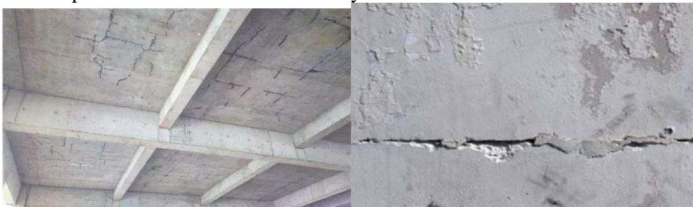
Fig.1 Cracks Caused by Temperature Factor
