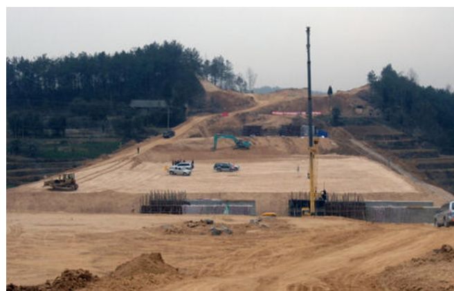
Fig.2: Waterproof Bonding Layer Construction
