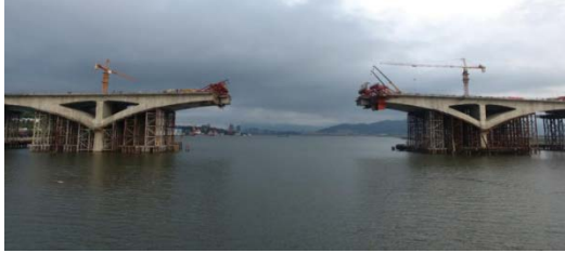
Fig.1 Main V-Shaped Structure of a Bridge
