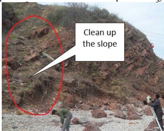
Fig.5 Cleaning area of Slope rock
