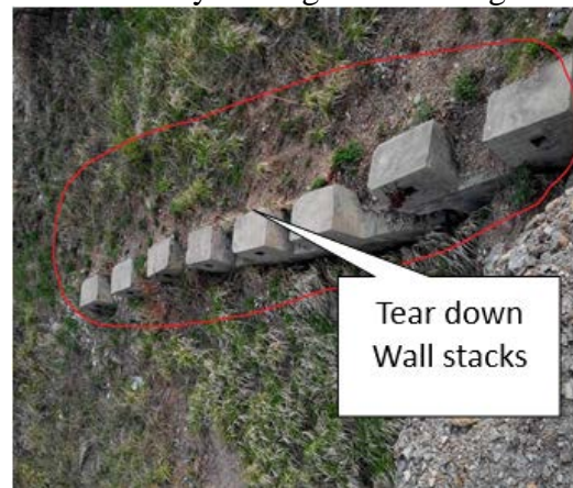
Fig.6 Tear down Wall stacks
