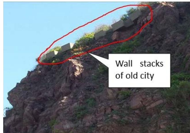
Fig.4 Wall stacks of old city
