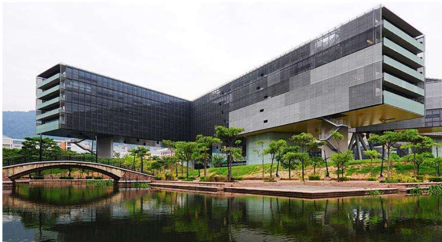
Figure 1 Green Building Representative Picture Source www.vanke.com
